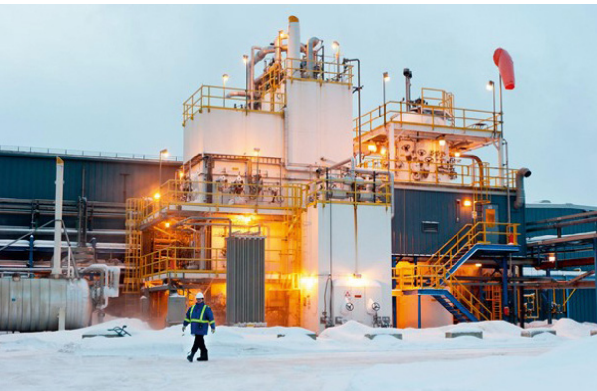
The Bécancour plant in Canada, the world's largest proton exchange membrane electrolysis plant with a capacity of 20 megawatts, was commissioned in January 2021.
